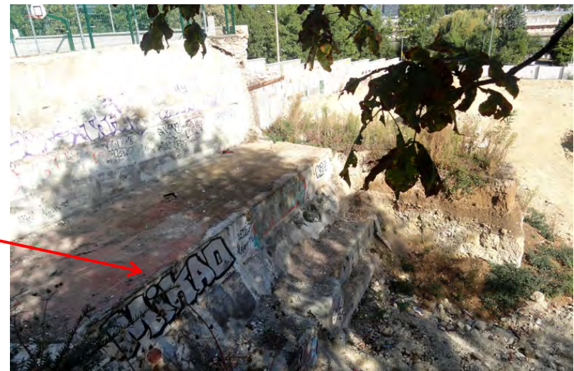
Demolished factory site
